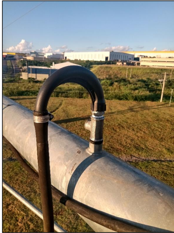
Figure 13 - Connection of the sprinkler elbow to the nipple.
