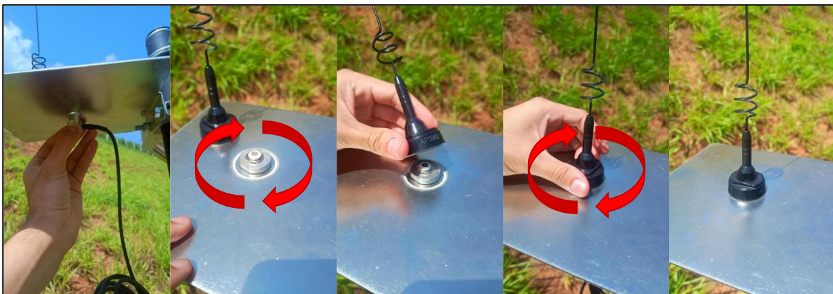
Figure 7 - Antenna Installation on the support.
