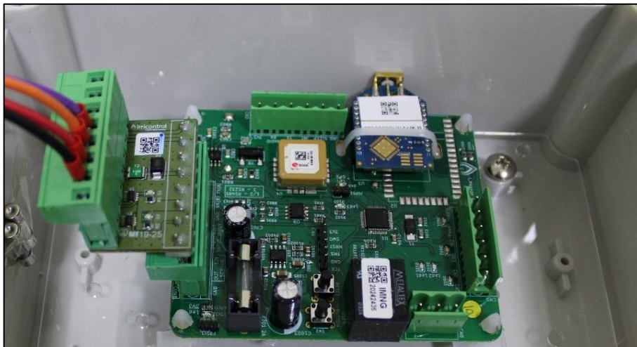
Figure 56 - Installation of the new Shield on the Imanage board.
