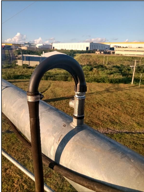
Figure 19 - Connection of the sprinkler elbow to the nipple.
