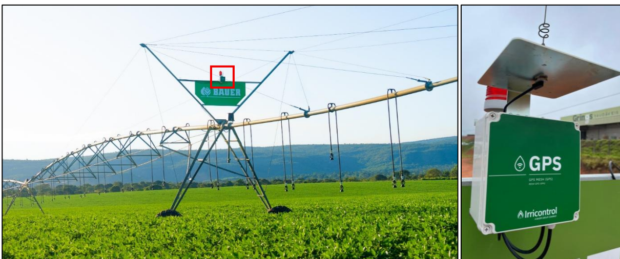
Figure 11 - GPS Installation on the Last Pivot Tower.
