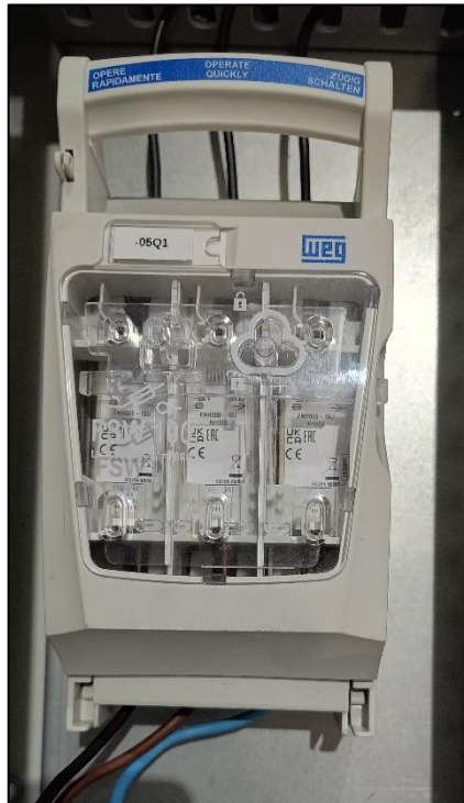
Figure 10 - The switchgear cover is in place.
