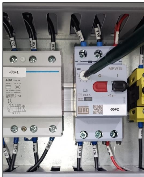
Figure 20 - Current limit adjustment.
